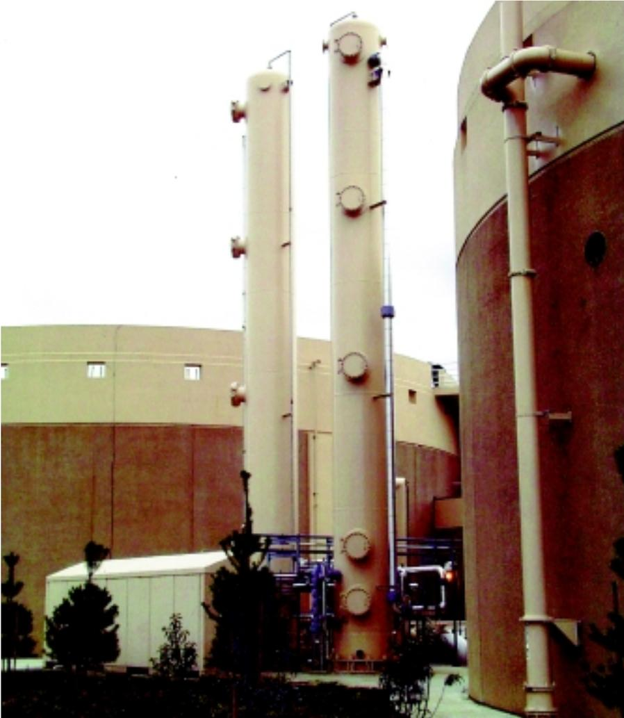
*Water scrubbing of carbon dioxide and hydrogen sulphide is often applied in Sweden, France and the U.S.A. The process is especially simple and usefull in sewage and industrial waste water treatment plants where the water does not have to be regenerated and recycled. The picture shows the Renton plant (Seattle, U.S.A.) with a capacity of 4.000 nm<sup>3</sup> per day.*
