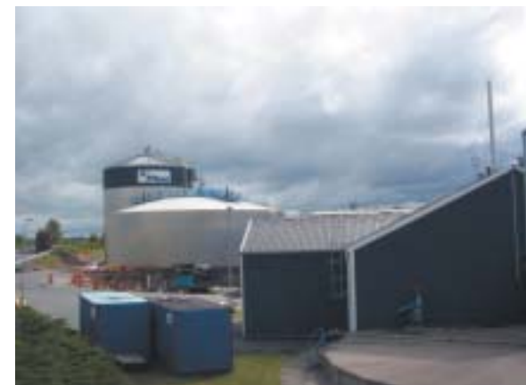
Manure and waste from the food industry is digested in Kristianstad, Sweden. The biogas is used for vehicles.
