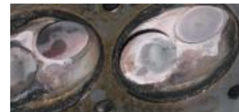
Siloxane deposits at the cylinder of a CHP engine
